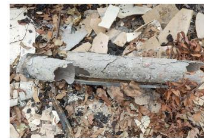
Figure 7 Fire damaged asbestos cement flue.
